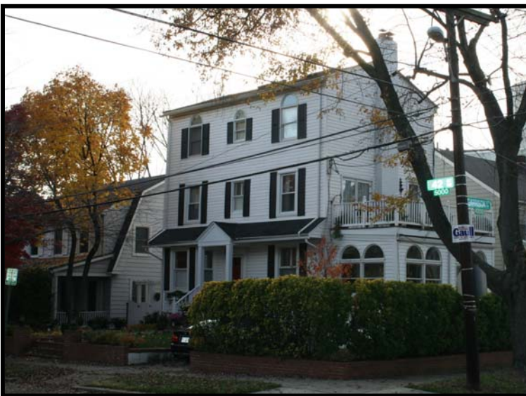
Loss of Character-Defining Features: Addition of second and third stories
